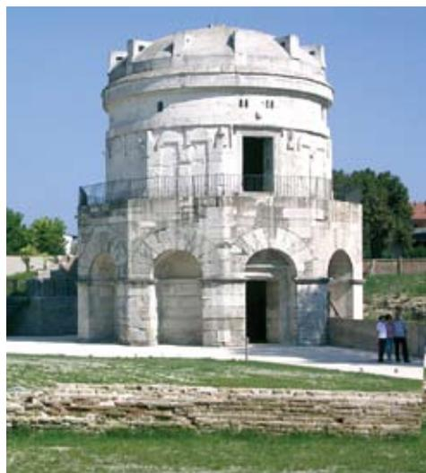
**Theodoric's Mausoleum** Entirely made of Istria stone on the model of more ancient sepulchres, the Mausoleum was built in 520 A.D. by order of Theodoric. A single block of Istria stone covers the structure, measuring 10m in diameter and weighing 300 tons. The decorations in the king's tomb were gradually removed along the centuries. In its interior, there is a circular porphyry tub in which Theodoric was supposedly buried.
